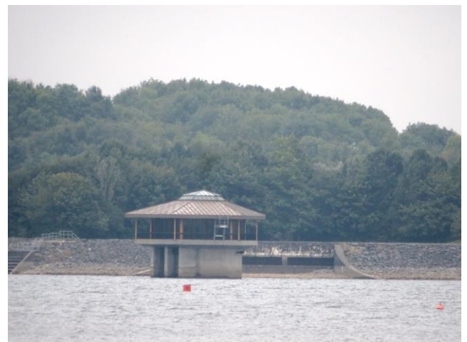
A closer view of the reservoir control tower and the dam wall
